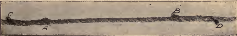
Fig. 8. The Repair Completed
